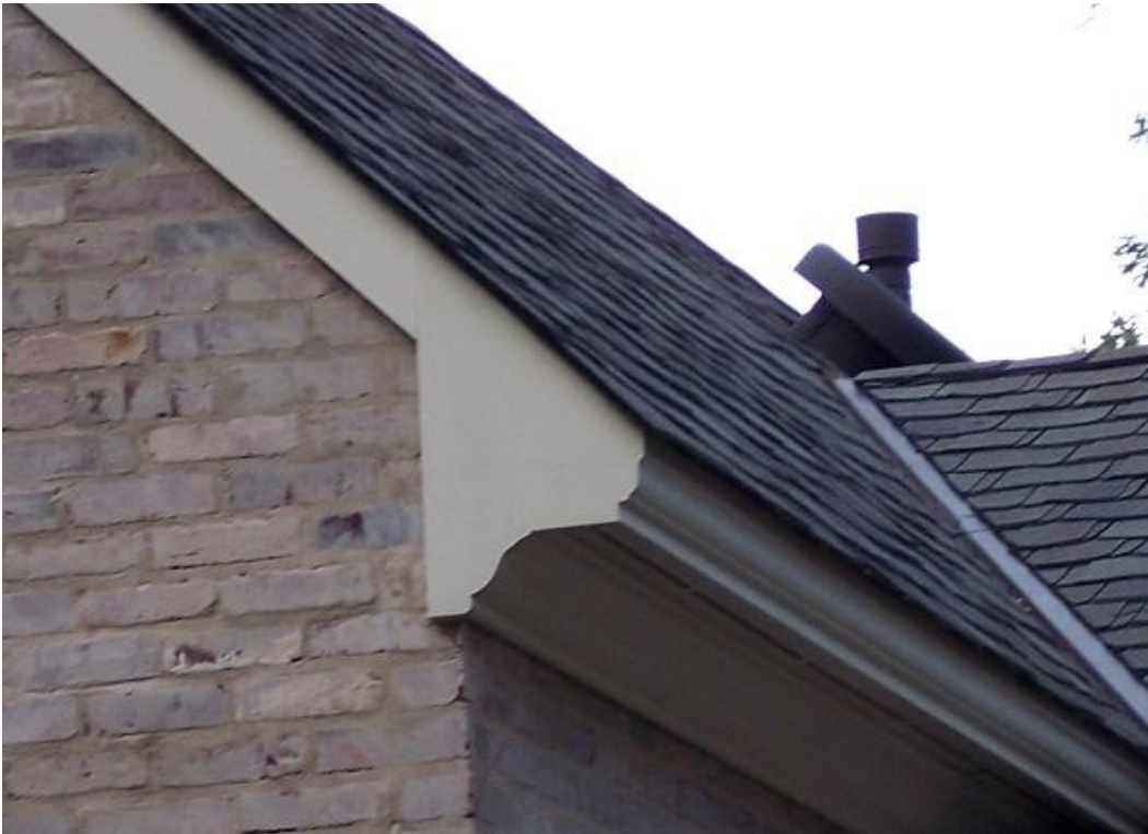
PROFILE - Flush Rake with decorative cornice end board as a molding stop
